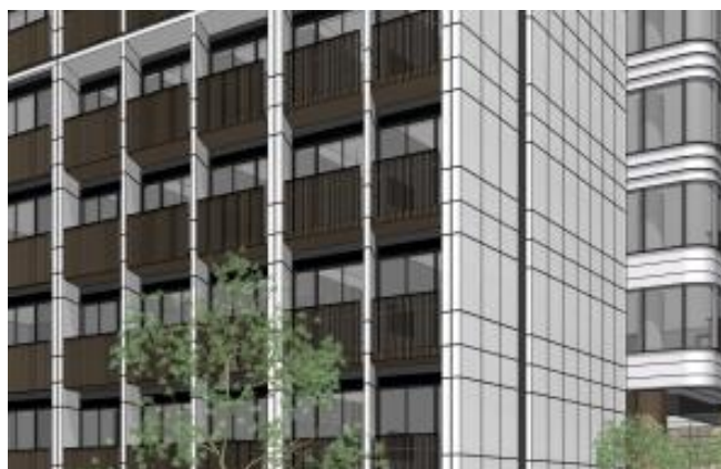
Figure 68 Precast walls form the western façade
